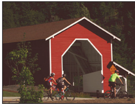
Office Covered Bridge - Kathy Baker
